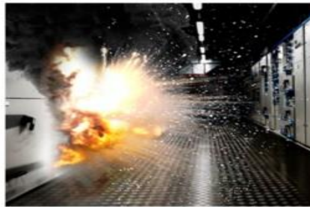
Arc flash - Typical ~ 12'000°C - Maximum 2,3 ~ 20'000 °C
